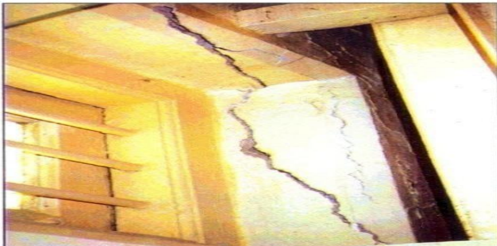
Fig -3 Crack in concrete due to corrosion of steel
