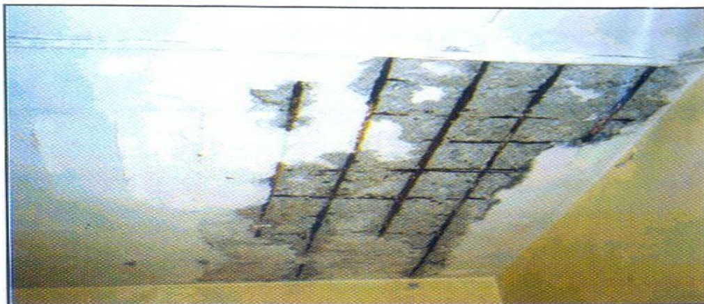
Fig 2 Corrosion of steel and Spalling of roof concrete on a slab
