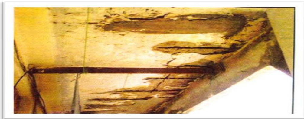
Fig- 1 Corrosion of steel and Spalling of concrete in a RCC canopy.
