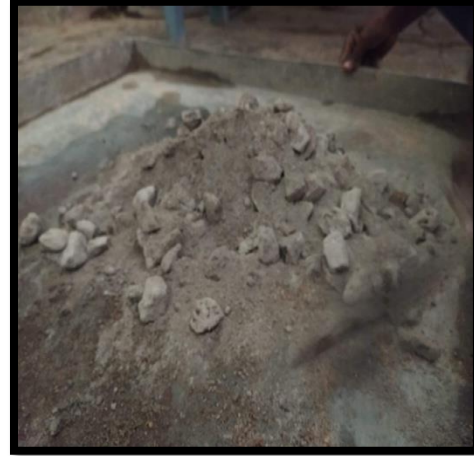
Fig. 2 Dry mixing of concrete
