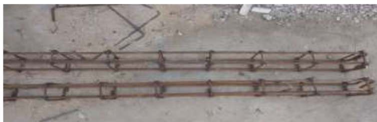
Fig. 1. Steel Reinforcement for the beam
