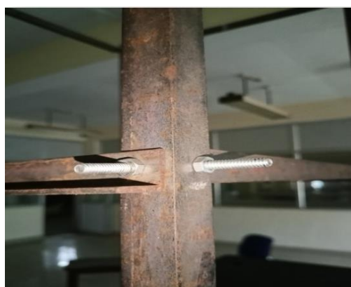
Figure 3. STEEL FRAME BOLTED JOINTS
