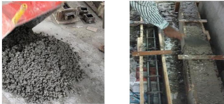
Figure 8 Filling cement to steel structure
