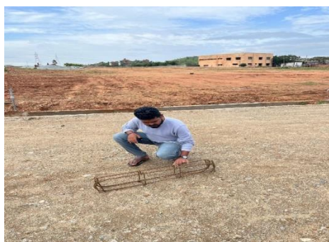
Figure 6 beam design using steel and binding wire
