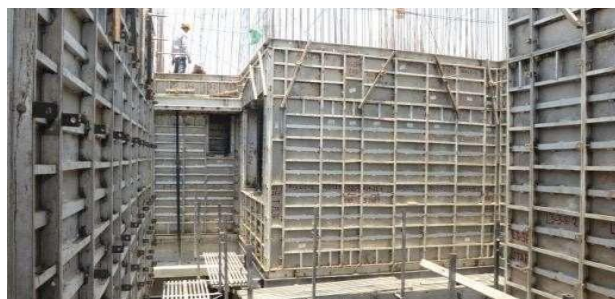
Fig 1.1 CONSTRUCTION USING MIVAN TECHNOLOGY
