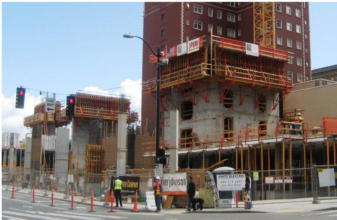
Figure 1: Construction of concrete walls for a high-rise apartment building. The structural system has two individual walls, at left, and a concrete core, at right (courtesy of KPFF) [17]
